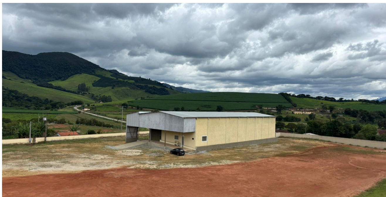
Project facility in Natércia. MBR photograph.
